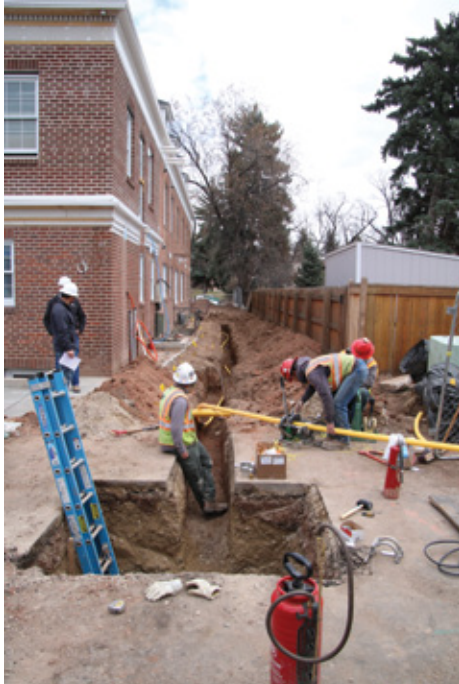
A new 2" gas line had to be installed.
