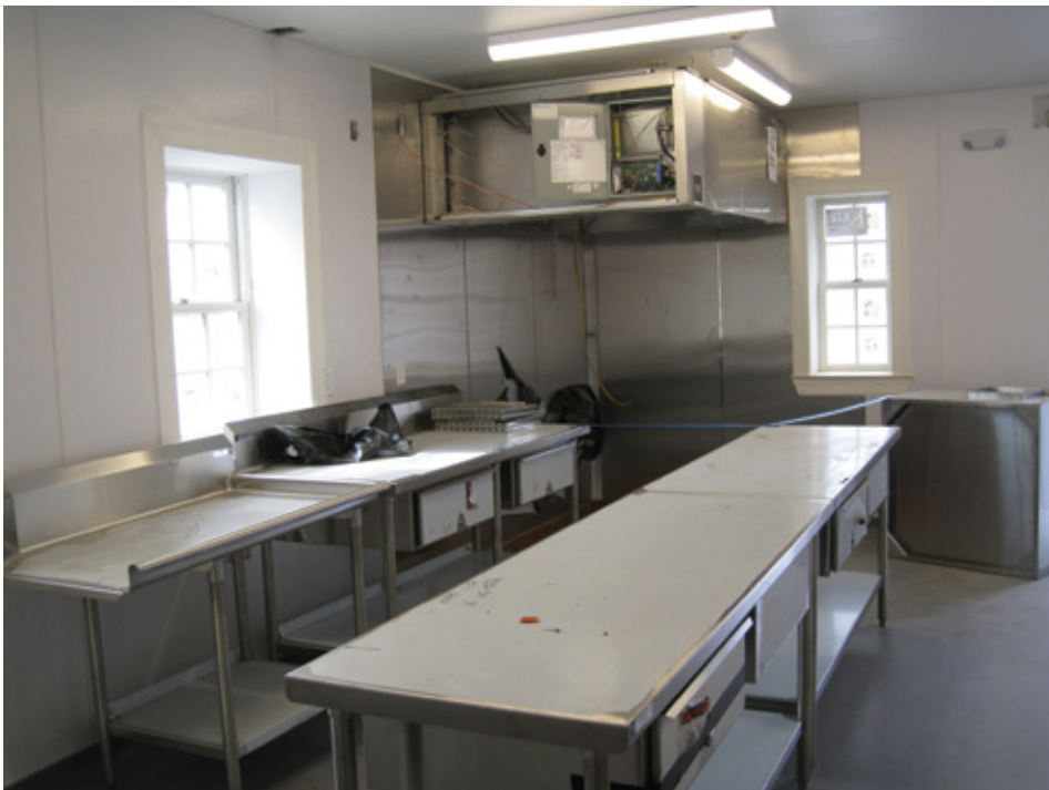
Kitchen is nearing completion.
